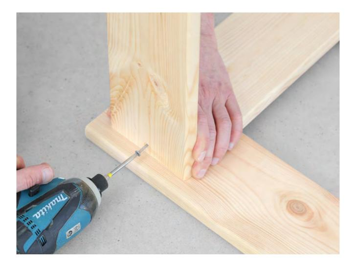
Make sure to align the planks before screwing. Use your fingers to feel the alignment.
