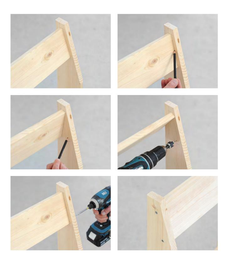
Rotate back rest in the position parallel to the angle. Mark the outline of back rest. Rotate the back rest out of the way to pre-drill the hole from inside for the position of the screw.
